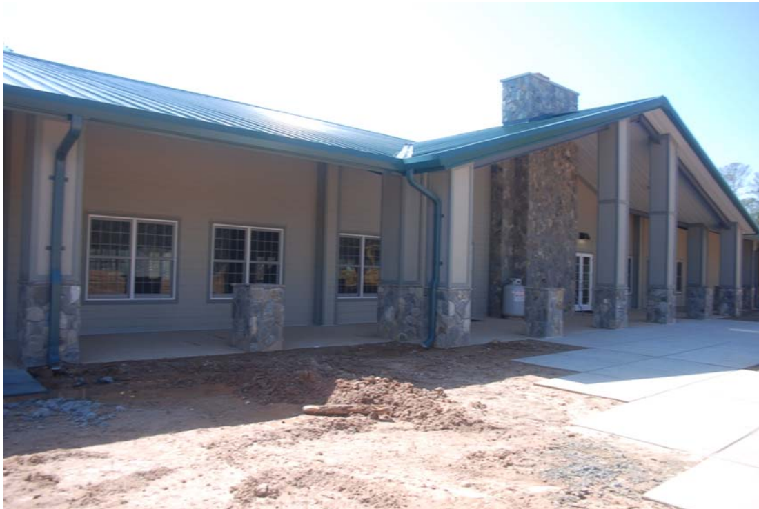
New Dining Hall will be in use during summer camp
